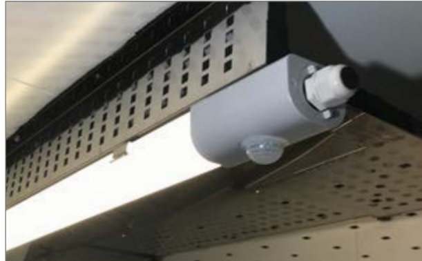
Lighting with motion sensor
